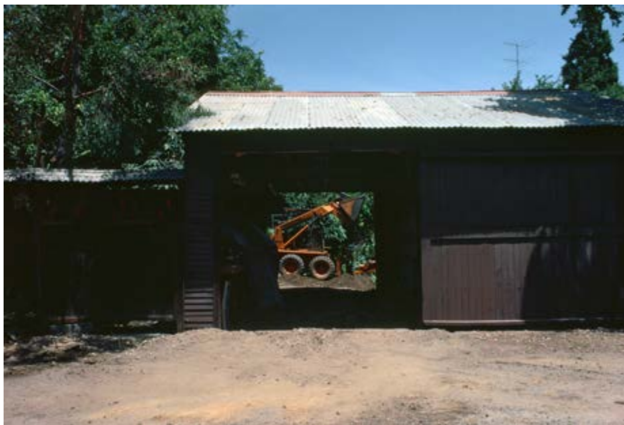
LEFT: Construction image of the T. House RIGHT: Sawyer Rose, Anne (2021)
